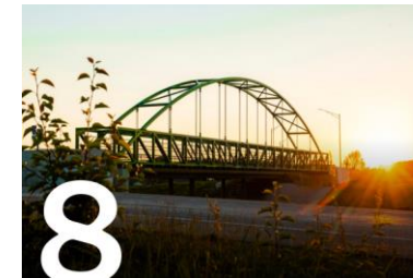
Finance and Infrastructure
